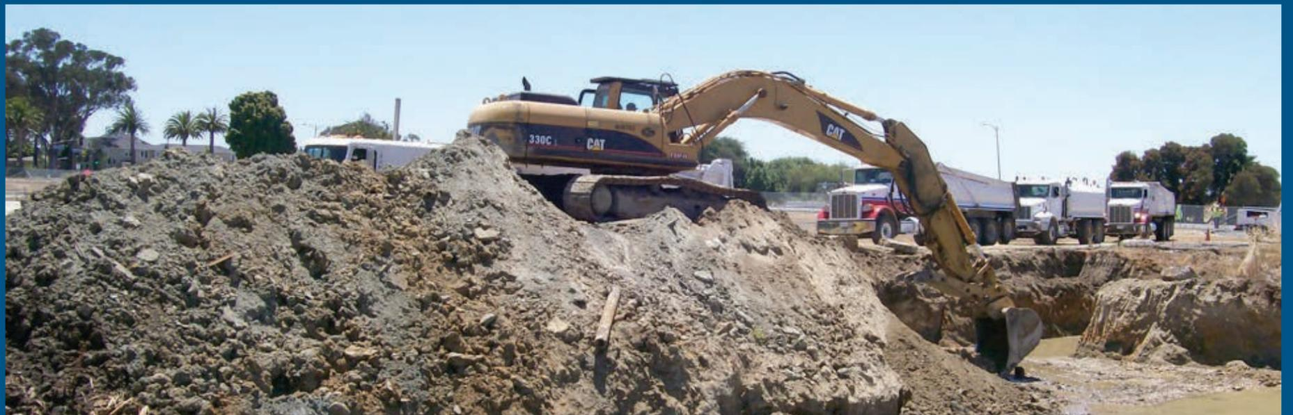
*An excavator removes impacted soils from the site of the former Building 637*
